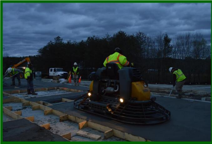
Once the walls are firm enough to support weight without making indentations, which is only about an hour after pouring, workers use a "riding trowel machine" to smooth the walls and ensure that they are exactly the same thickness at any given point.
