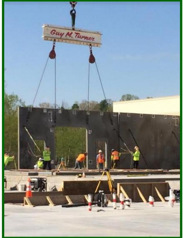
A giant crane lifts the wall panels one by one into place and holds them as workers secure them in place. The crane for moving the walls is so large that it arrived at MCA on four trucks, and it required a smaller crane to help assemble it.
