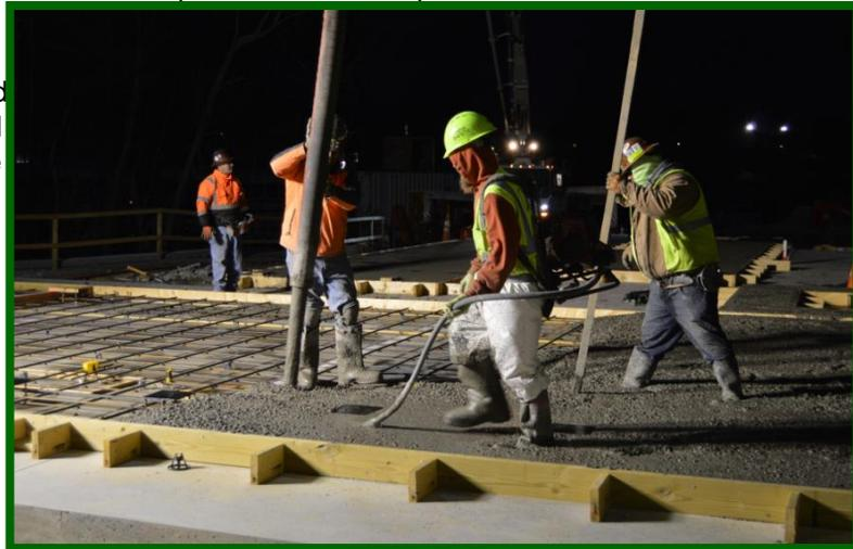
Finishers work during the night to create the walls. One person guides the pipe pouring cement into the wall forms, as another uses a vibrating machine to settle the concrete and remove air pockets.
