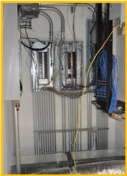
The photo above shows the electrical closet, the infrastructure hub for the new building. This is the location for electricity, voice, data, and HVAC to come "home" for control. Voice and data cabling is complete, and other wiring is well underway.
