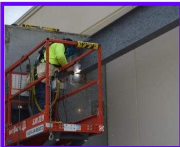
Left: The signed beam is welded into place. Right: the signed beam is adjacent to the existing building on the side nearest the back driveway.
