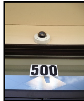
The security camera over the main front door captures images of persons approaching the door and traffic in the main parking lot.
